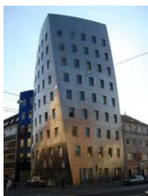
Slika 9. [7] Gehry-tower, Hannover, Germany.
